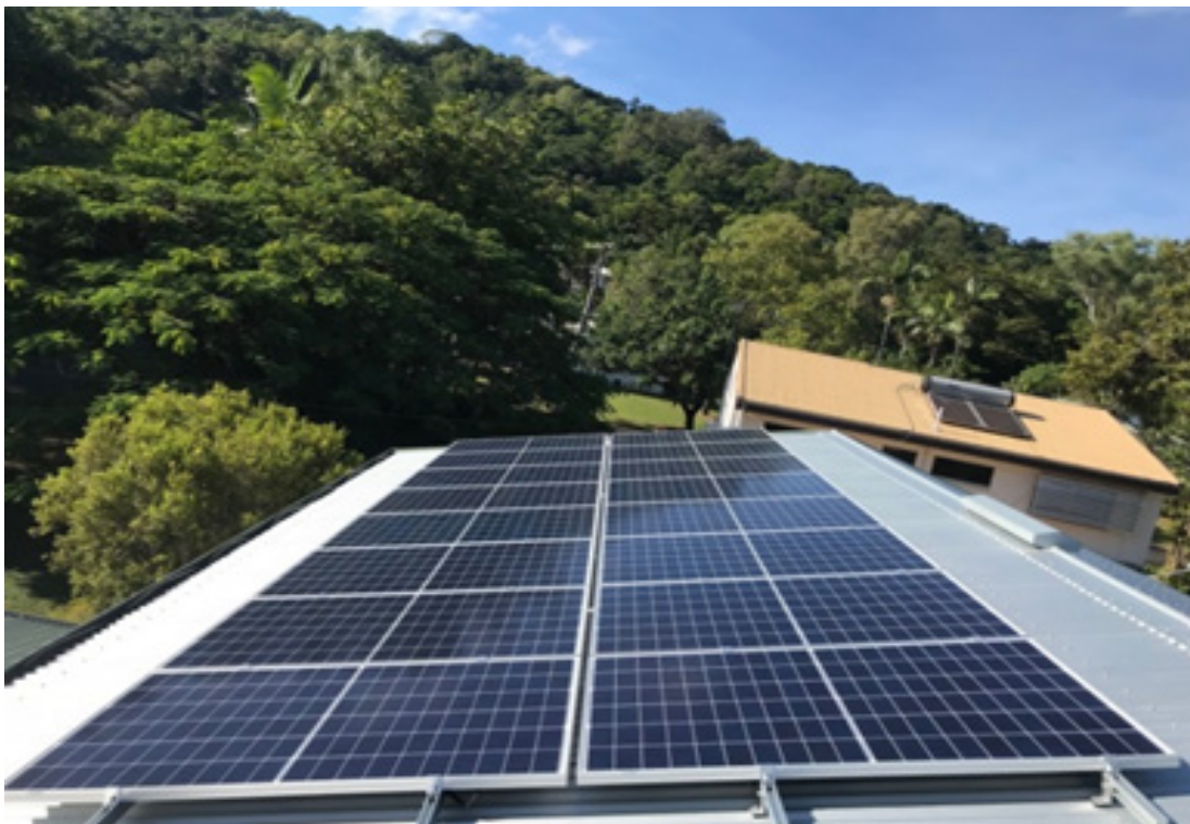
Panels installed at Simon Street Freshwater, Queensland
