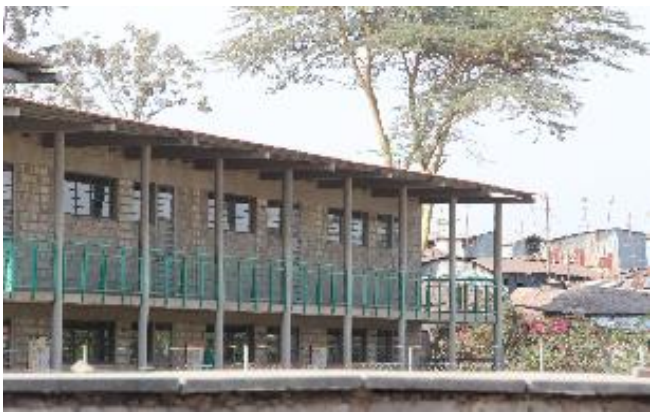
The newly built school at Lunga Lunga. St Elizabeth's was constructed by a group of German Entrepreneurs through the German Government.
